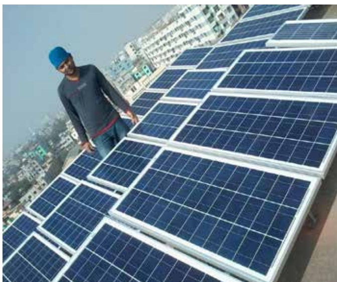
Solar system work
